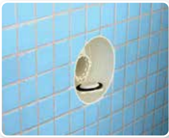
Remove Dress Ring Cover, open spring loaded port.
