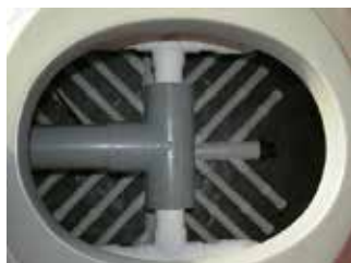
Lateral under drain system
